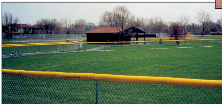
Safety takes effort: (above) Adding protective tubing to fence tops reduces risk of players being injured reaching for home-run balls; (top right) bleachers are more safe with handrails and back guards; (below) ball returns help get balls into play safely; (bottom) and safety bases reduce sliding injuries.
